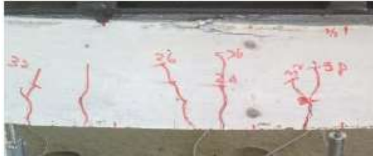
Fig 6. Shear failure of the tested beam
